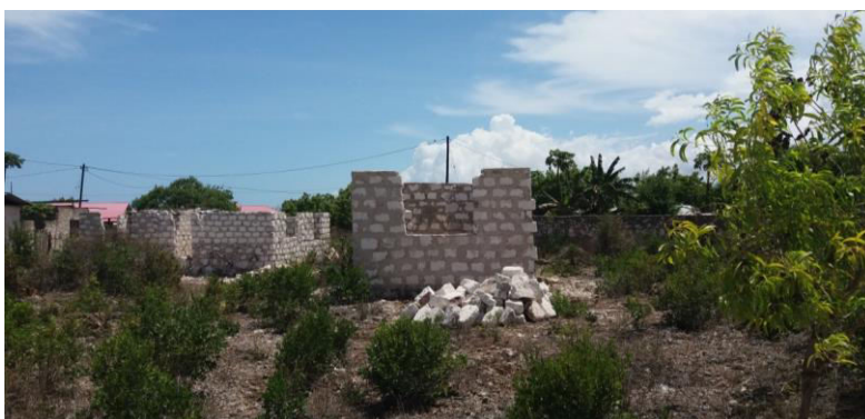
Figure 7: Some new houses built of stone bricks in Matemwe village.
